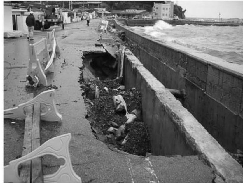
Figure 3. Wave overtopping (left) and resulting damage (right) in September 2007.
