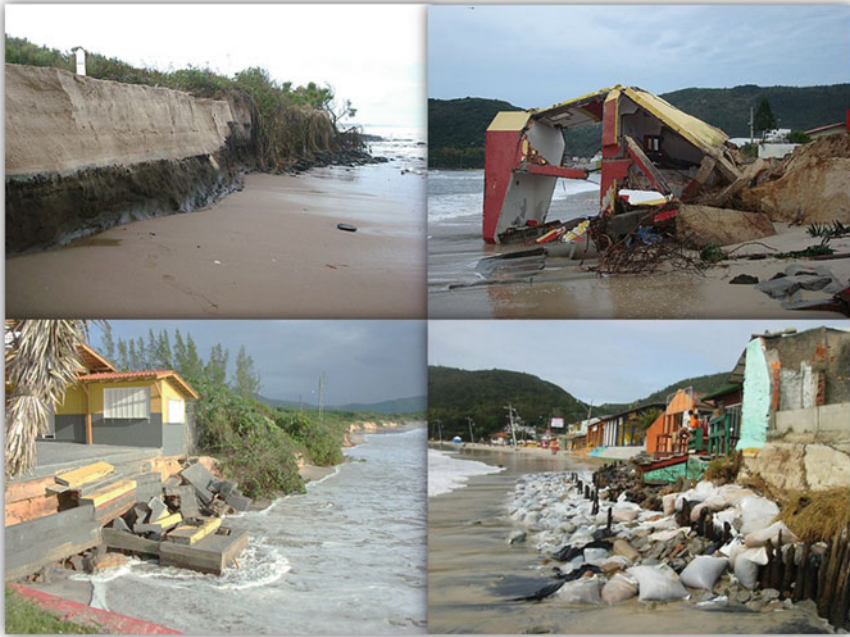
Fig. 16.4 Morphological impacts of an extreme storm event (April 2010) along the beaches of Barra da Lagoa and Moçambique (Photos by J. Bonetti)
